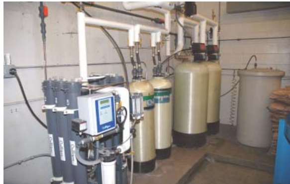
This is one of several incoming water treatment equipment stations located in the Cardiovascular Division of St. Jude Medical.
